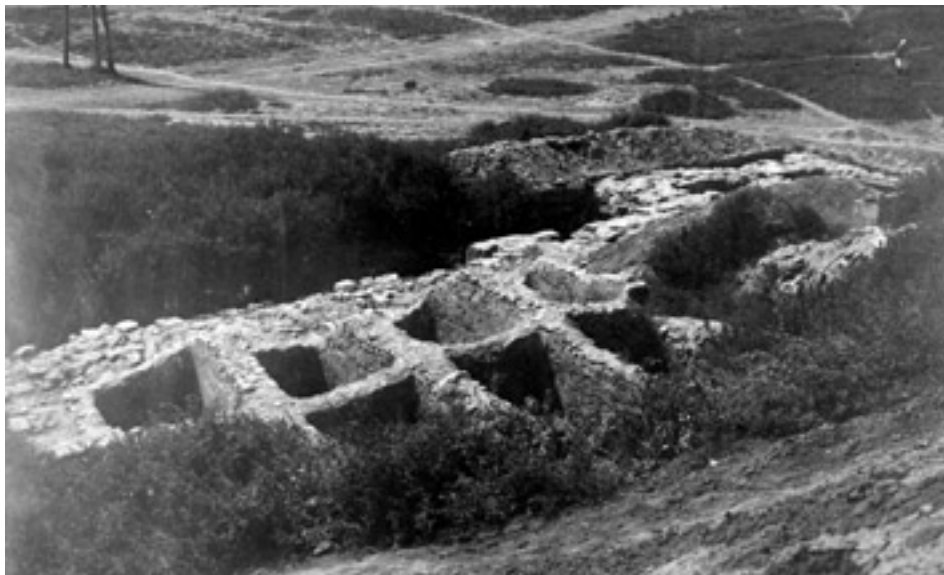
Fig. 6. The largest salting installation with originally 16 vats located just inside the southern wall. The vats had a capacity of 155 m 3 (courtesy of the Photo Archives of IIMK RAN).
