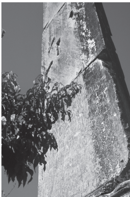
Fig. 23. Detail of the monument, showing recesses in the side of the vertical stone face, intended for lead cramps to hold standing bronze figures. Similar recesses are cut into the top surface of the base (author's photo).
