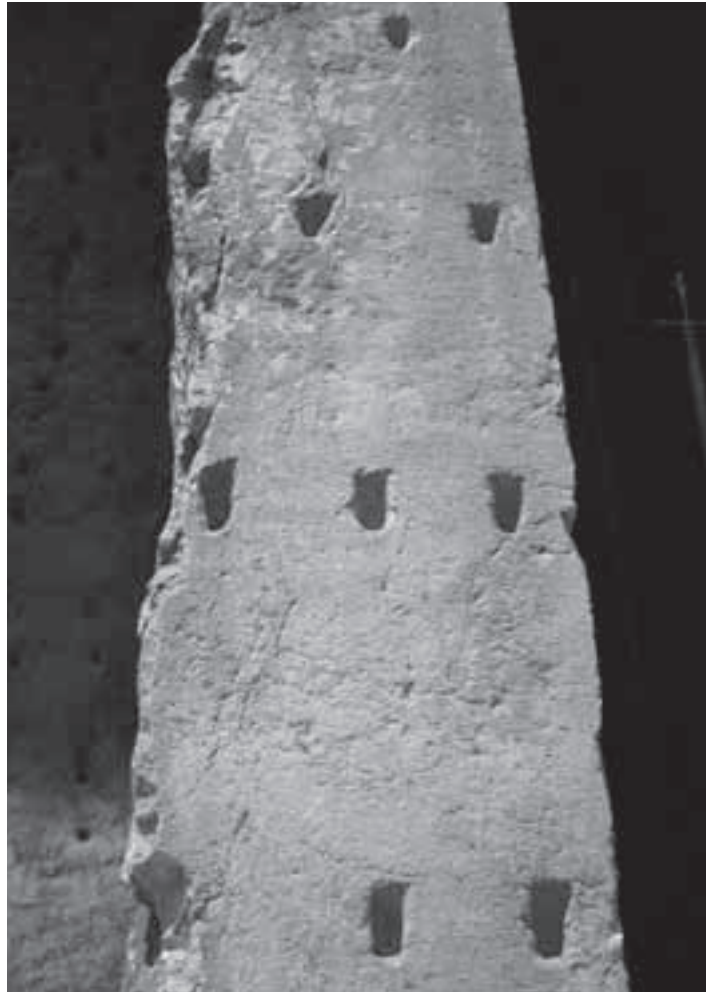
Fig. 3: Cuttings for fastening architectural details on the front of the ante on the "unfinished tomb".
