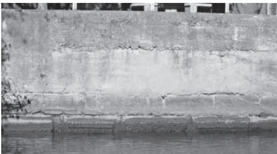
Fig. 20. Inscription blocks built into the foot of the Roman bridge that is now incorporated into the water regulator.
