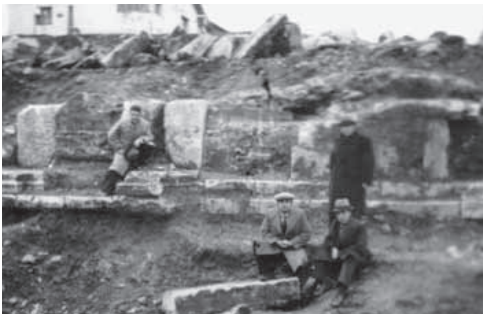
Fig. 19. An old photograph of ruins from the vicinity of Hamamtepe or Hamamtepe itself during the construction of the water regulator (from the archive of M. Cinlioğlu).
